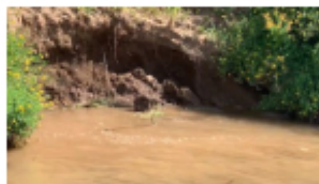
Shoreline bank erosion
